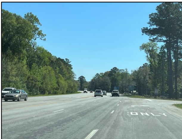
Looking east towards proposed driveway location along SC 170
